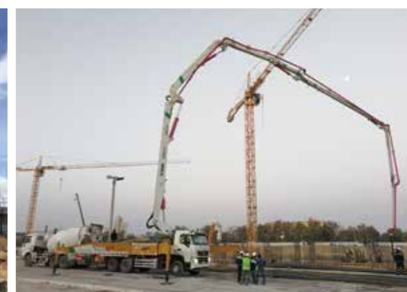
徐工泵车助力乌兹别克斯坦建设 XCMG boom pump is working in Uzbekistan
