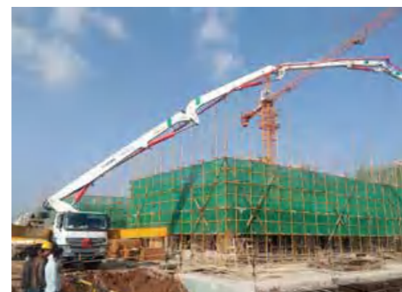
徐工HB52V泵车云南施工 XCMG HB52V boom pump is working in Yunnan
