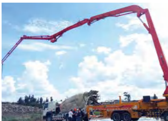
徐工泵车助力埃塞俄比亚建设 XCMG boom pump is working in Ethiopian construction
