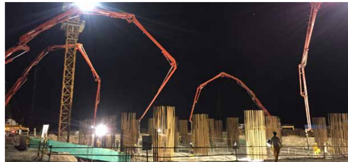
四蛟龙齐助尼日利亚建设 Four boom pump are cooperating like dragons in Nigeria
